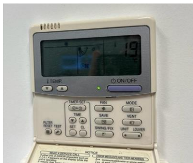
Figure 10 – Console for individual control in the room (remotely monitored to control the set-point)
