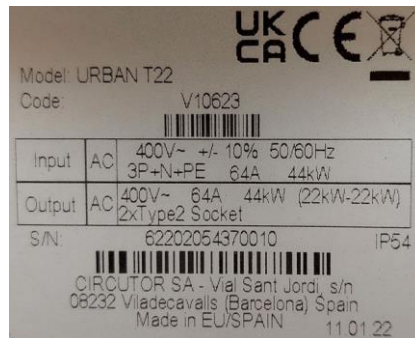
Figure 9 - Characteristic sheet of EV charger from Computer Science Faculty
